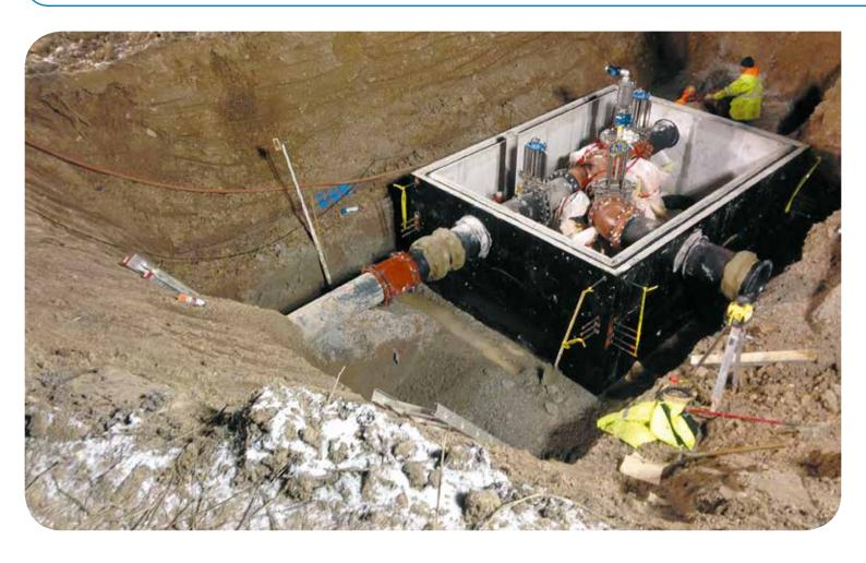
Making a connection in the middle of the night at -20 °C is not easy. Especially if you have to connect HDPE SDR11 to HDPE SDR 32,5 you are in a world of trouble. But not if you use the MULTI/JOINT® 3000 Plus.
